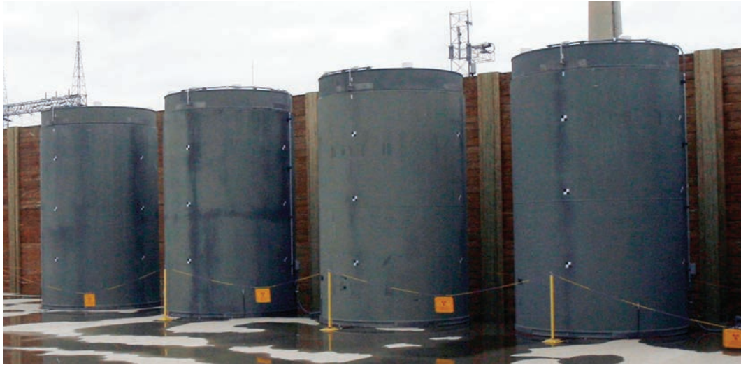
After about five years in a cooling pool, spent reactor fuel can be transferred to dry casks like these, which do not need electric power to keep the fuel from overheating.
