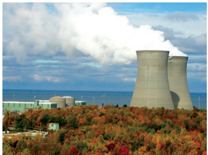
Inspections at the Perry plant in Ohio illustrate a successful oversight process.
