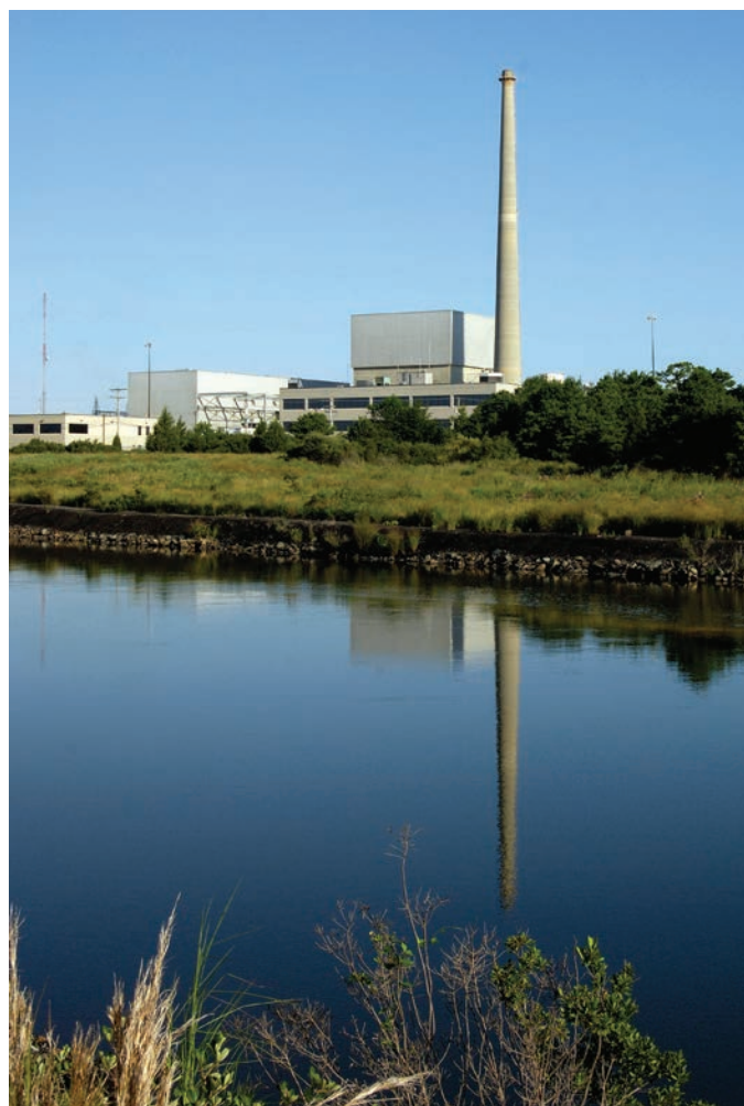
Oyster Creek nuclear plant in New Jersey lost offsite electrical power following Hurricane Sandy.
