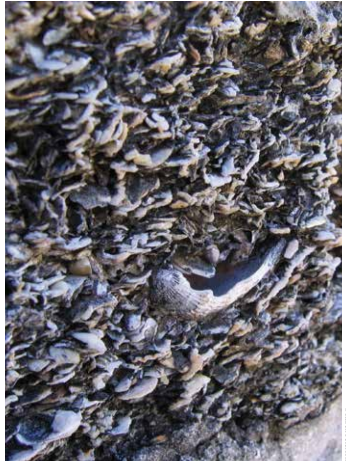
This close-up illustrates the coquina construction used at Castillo de San Marcos. The ocean's constant pounding meant the wall required reinforcement, and the National Park Service has taken steps to create a living seawall to protect the historic coquina wall. 257
