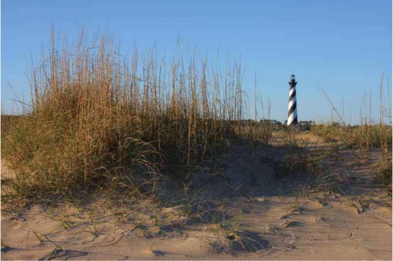
The Cape Hatteras Lighthouse, a witness to Spanish and pirate ships, Civil War battleships, and German U-boats, was moved inland nearly 3,000 feet to escape relentless sea level rise and coastal erosion—at a cost of approximately $11 million. 203
