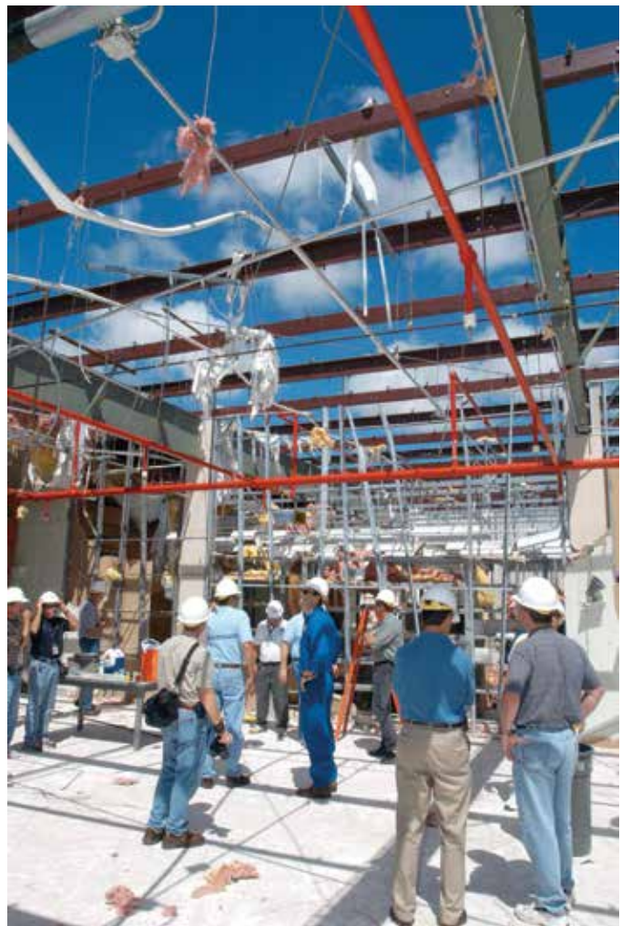
Members of a hurricane assessment team observe the damage to the roof of the Thermal Protection System (TPS) Facility at Kennedy Space Center after Hurricane Frances (2004). The facility, which created the TPS tiles, blankets, and all the internal thermal control systems for the space shuttles, was almost totally unserviceable after losing approximately 35 percent of its roof. 168
