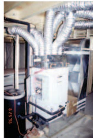
A properly sized HVAC system with centrally located ducts eliminates heat loss.
