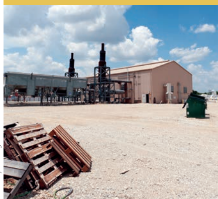
Hog Branch compressor station, Dish, Texas
