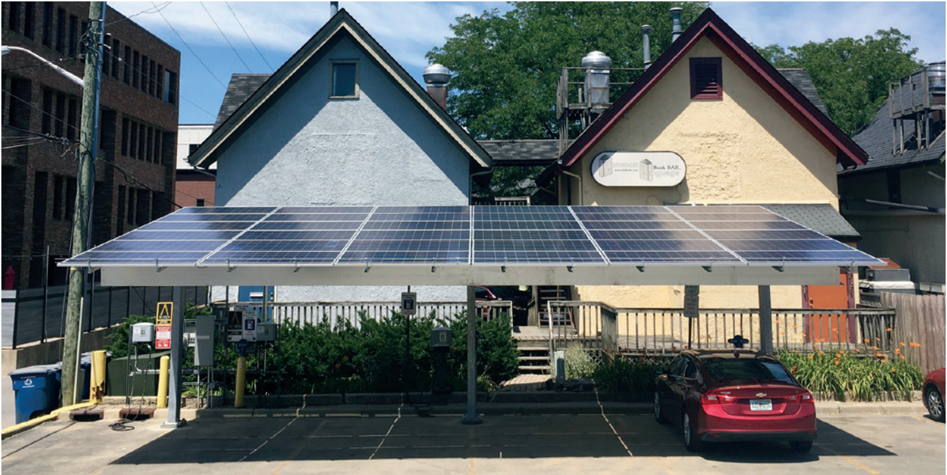
A solar carport sits above electric vehicle charging stations in a parking lot in Ann Arbor, Michigan. Carports and solar canopies can be installed on already developed land parcels, providing shade while also generating clean electricity.
