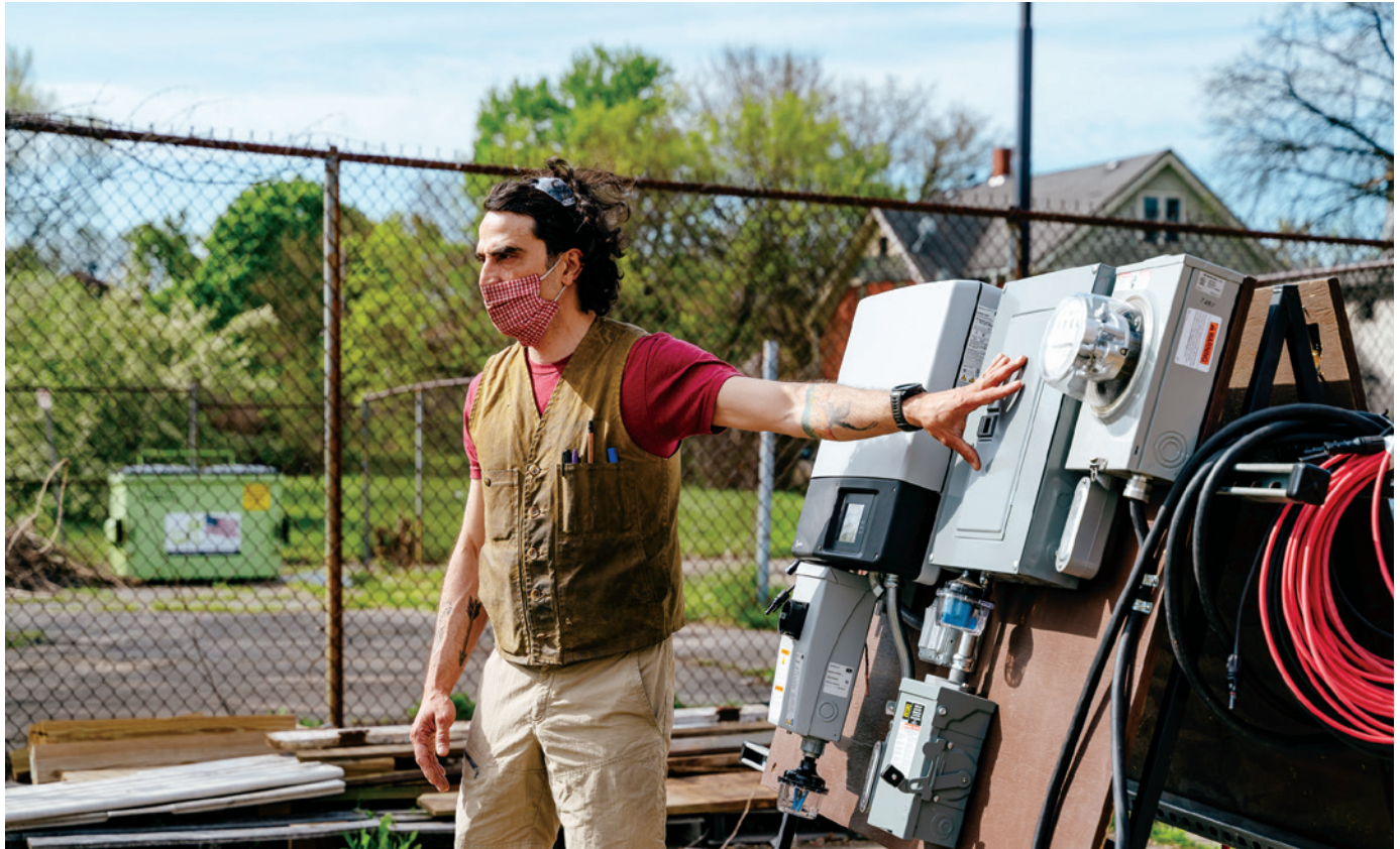
At a solar training at Parker Village in May 2021, Highland Park residents learn about how rooftop solar projects connect to a home's electricity meter.
