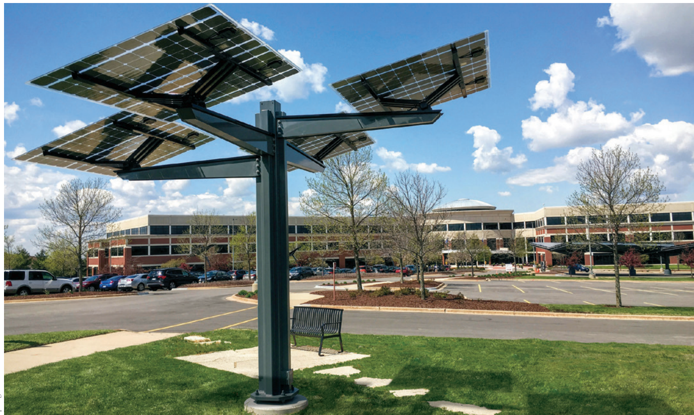
Solar trees, like this one in Madison, Wisconsin, allow for distributed solar generation in open areas such as parks while preserving the land underneath for other uses.
