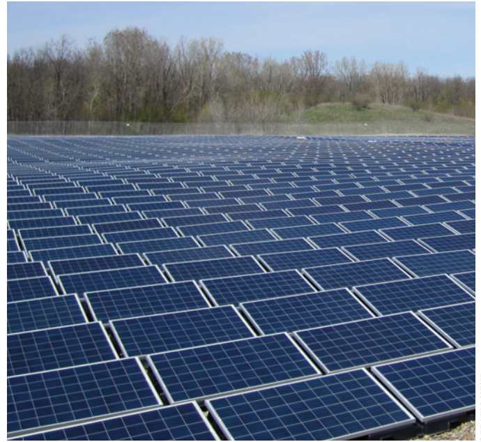
Disturbed lands such as closed landfills can be excellent locations for PV projects. In Michigan, solar panels on a 100-year-old former landfill are supplying electricity to the nearby city of Eaton Rapids.
