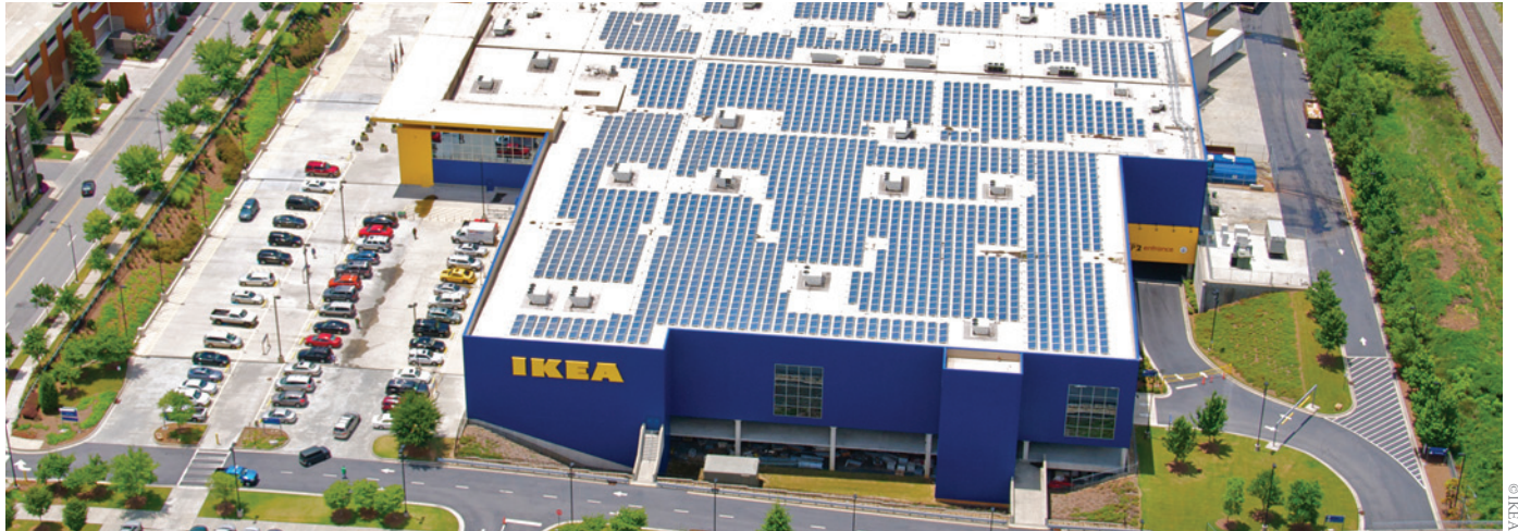
Many large companies in the United States have “gone solar.” IKEA has rooftop solar on 89 percent of its stores, including this store in Atlanta, GA, and meets more than one-third of its electricity needs with renewable generation (IKEA 2013; SEIA and Vote Solar 2013). Walmart has more than 200 PV systems, amounting to 89 MW of solar generation capacity (SEIA and Vote Solar 2013).
