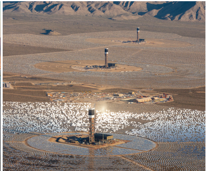
CSP comes in different forms, and involves different options. Left: The 250 MW AC Solana parabolic trough project outside Phoenix, AZ, is one of several CSP projects in the United States that incorporate energy storage. Right: The 390 MW AC Ivanpah power tower project, located next to a golf course and highway near California's border with Nevada, cools its electricity-producing steam with air instead of water, cutting water consumption by 90 percent or more.
