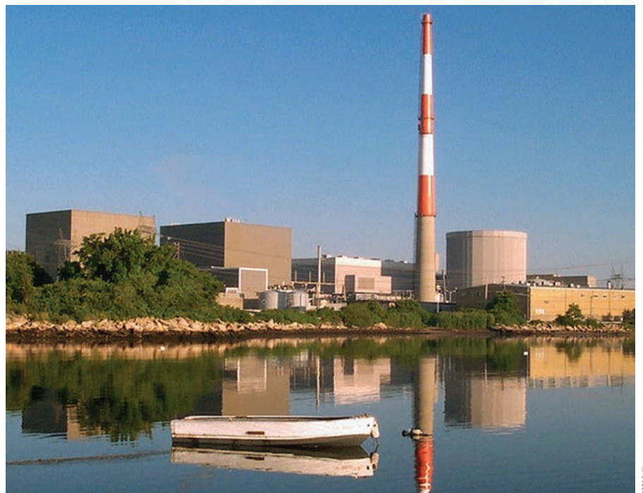
The Millstone Power Station in Waterford, CT, which experienced two self-inflicted near misses in 2014 when recent maintenance and modifications introduced problems that reduced safety margins.
