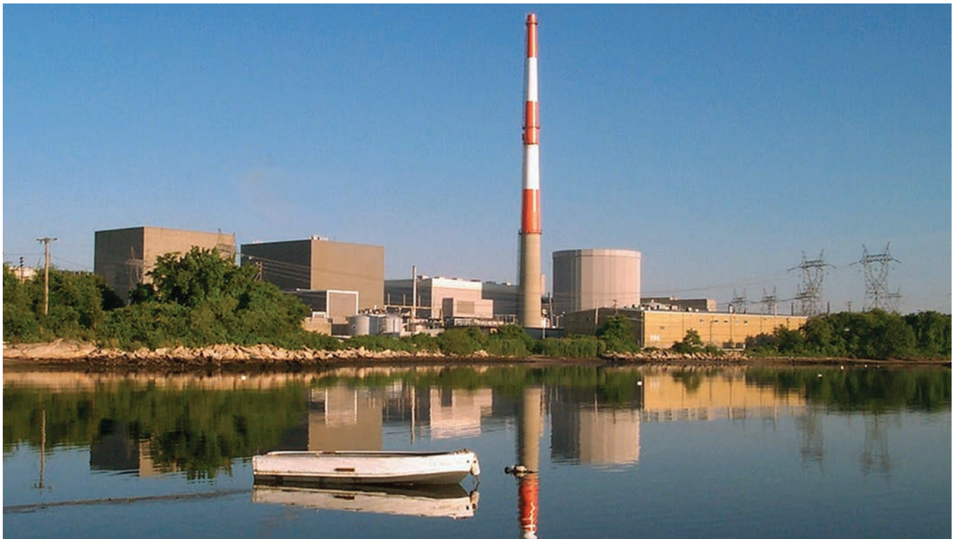
The Millstone Power Station in Waterford, CT, which experienced two self-inflicted near misses in 2014 when recent maintenance and modifications introduced problems that reduced safety margins.
