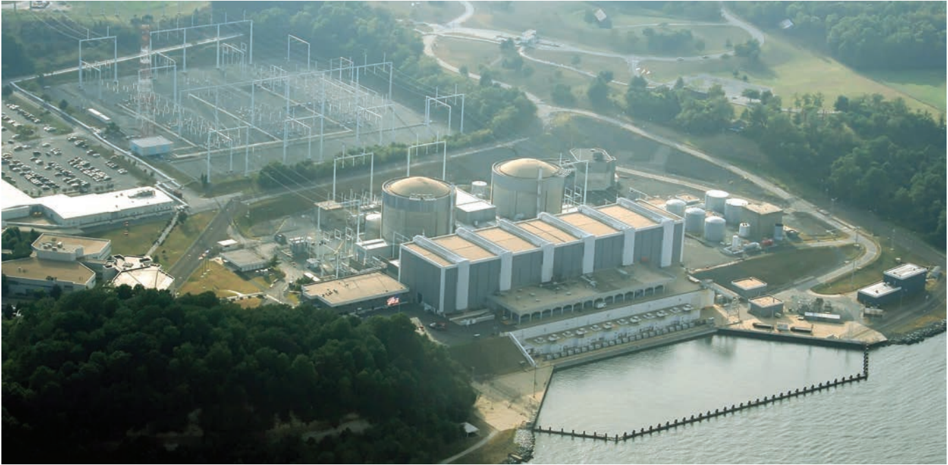
The Calvert Cliffs Nuclear Power Plant, where water leaked in during a winter storm to short out electrical circuits and force both reactors to automatically shut down.
