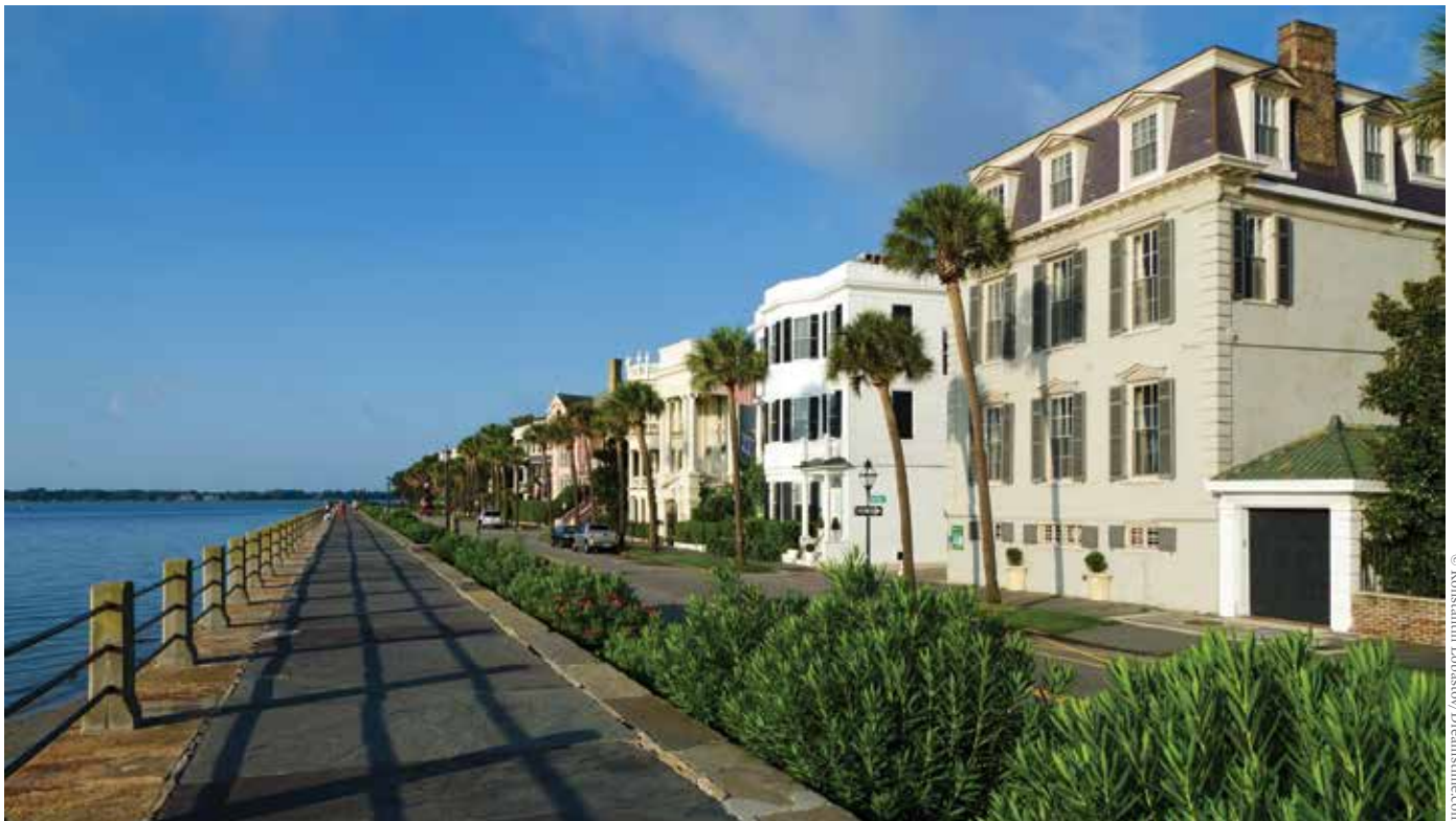
Charleston is at risk from hurricanes, sea level rise, and accompanying increases in tidal flooding. The city's historic Battery, a defensive sea wall and promenade, is vulnerable to major storms. Tidal flooding is routine today and projected to worsen as sea levels rise.
