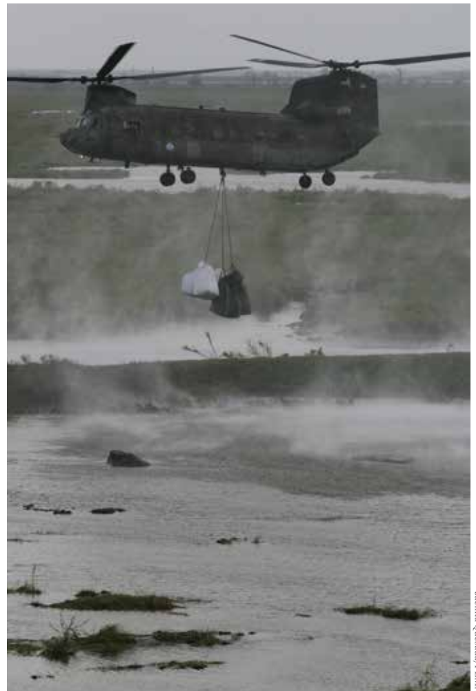
In the wake of Hurricane Gustav, a U.S. Army helicopter drops sand bags onto a broken levee in Plaquemines Parish, much of which lies below sea level and is particularly vulnerable to sea level rise and coastal flooding.
