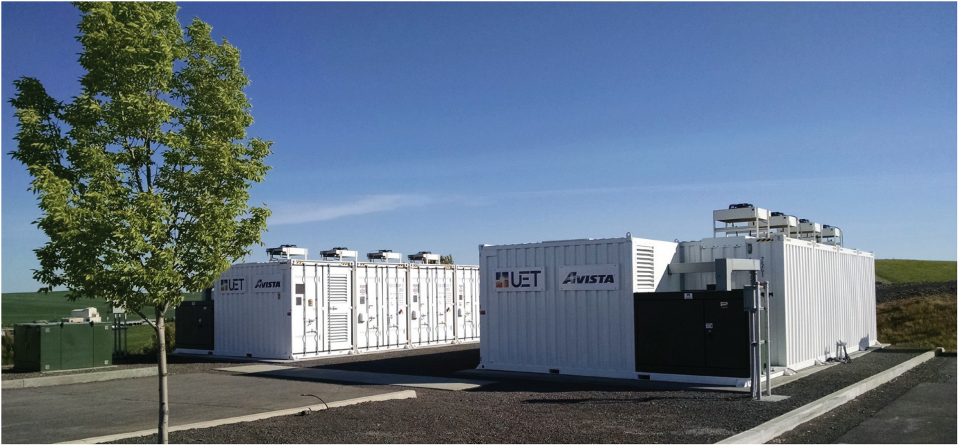
A 1 MW vanadium flow battery installed in Pullman, Washington. Advanced energy storage will play a key role in the modernization of our nation's electricity grid. Energy storage enables the integration of renewables, improves the grid's operating capabilities, enhances reliability, and provides backup power during emergencies.
