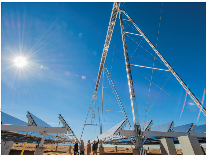
Funded partially by the Department of Energy, AREVA's solar team and Sandia's molten salt technology experts have developed an innovative approach to energy storage.
