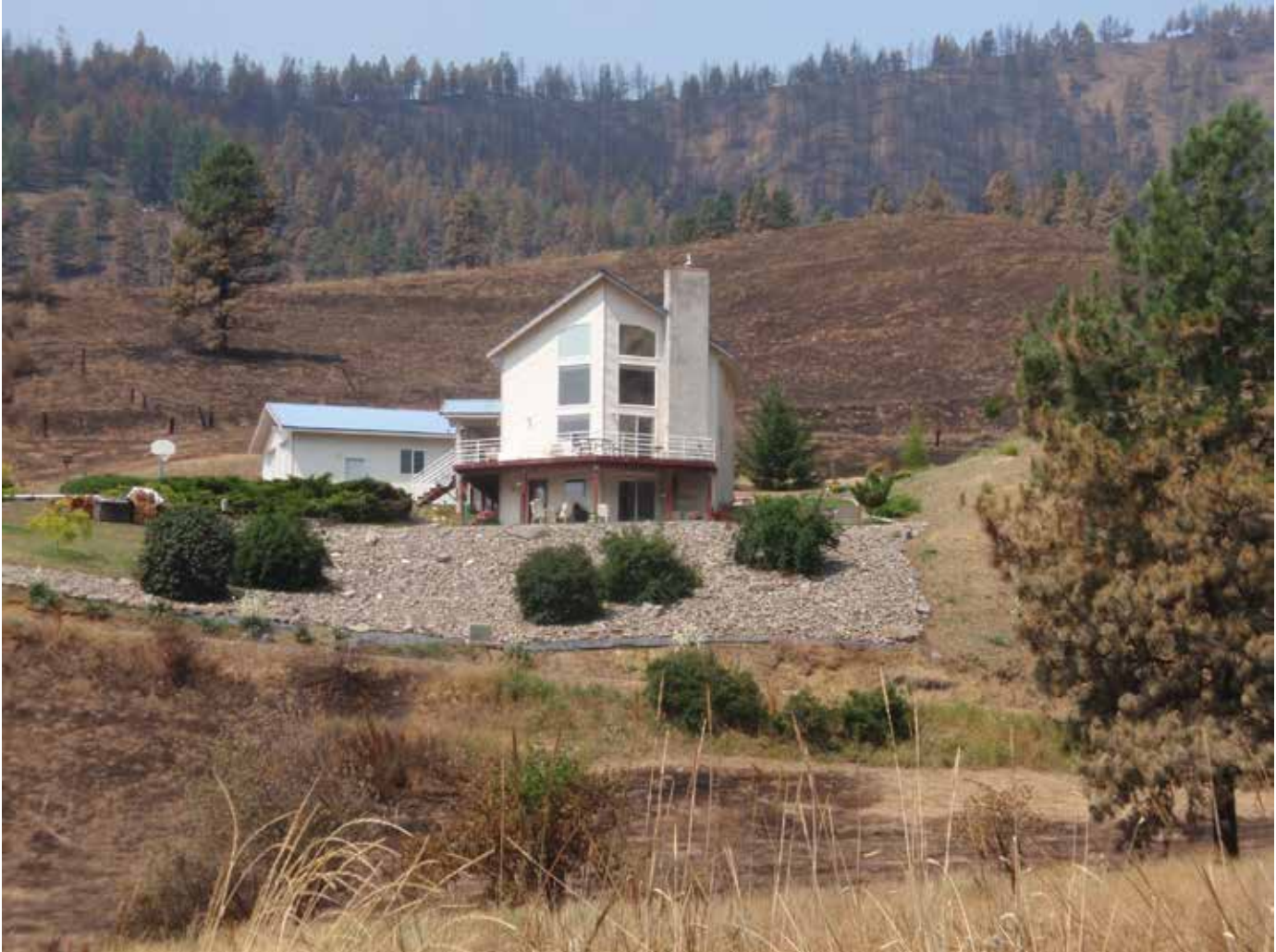
Homeowners who live near wildfire-prone forested areas can take steps to reduce their risks by investing in fireproofing measures. This homeowner has created a defensible space around their home, with no large trees in a wide perimeter around the home. This helps reduce the risk of fire spreading from forests to homes and also gives firefighters space to fight the fire.
